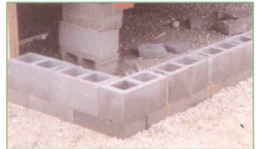
Mason Bond® was applied to vertical and horizontal surfaces of the base course.
