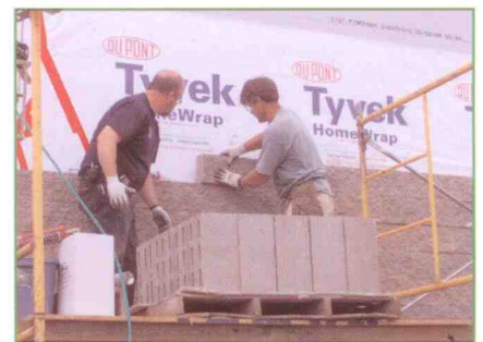
Owners cut over one-third off the cost - over $30,000 - by using Mason Bond™ adhesive instead of mortar on the Ozone Action City project.
